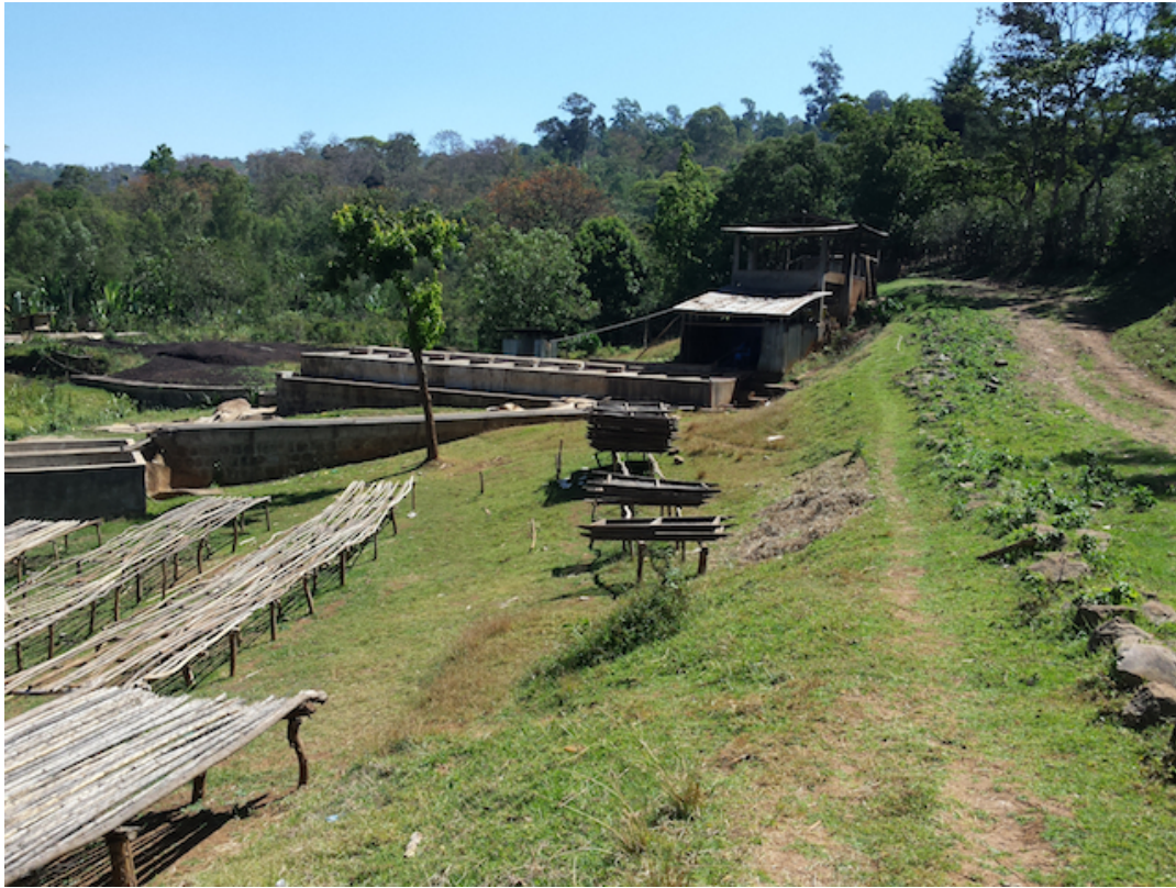
Figure 1. Typical coffee processing (wet) facility, Yirga Chefe, Ethiopia. Water is pumped from surface streams at base of slope for processing. Liquid and solid wastes are placed in excavated lagoons near waterways down slope of processing operation.
