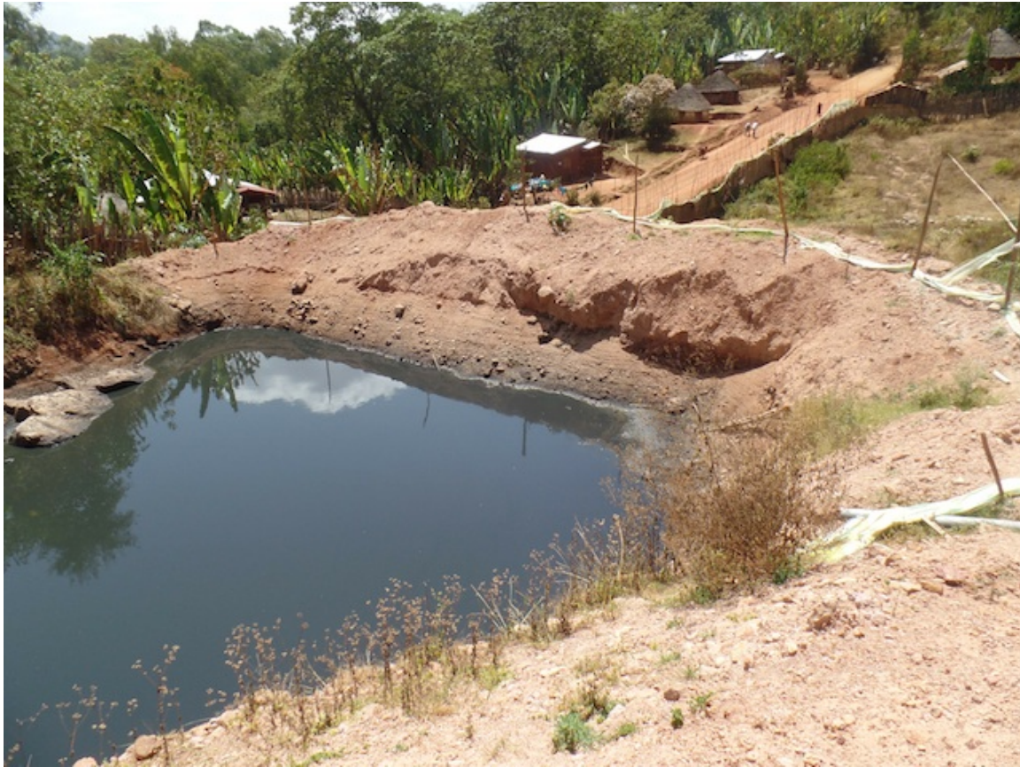
Figure 3. Liquid waste lagoon with processing wastes, Yirga Chefe region, Ethiopia. Poorly constructed waste lagoons threaten surface waters and nearby communities.
