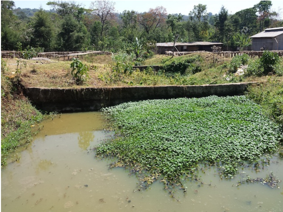
Figure 4. Multi-stage liquid waste lagoons can utilize photosynthesizing plants and gravity-based methods to oxygenate waste waters.
