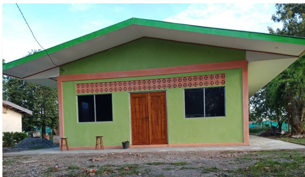
Auditorium funded by SEFOPE. Photo by CRS F2F Staff.
